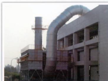
Waste gas treatment system with dust collector
